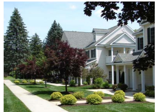
Pedestrian oriented scale, continuity of treatment including front porches, and roof design that adds visual interest, with integrated sidewalks and landscaping. Buildings overall contribute to surrounding area as a whole.
