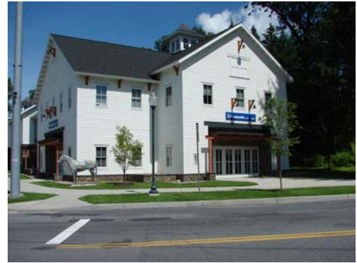
Two story building illustrating appropriate site layout, treatment and fenestration. Includes vertical alignment of windows.
